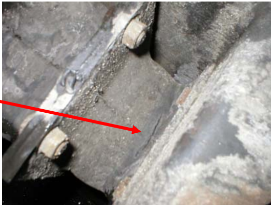
Fig. 3. Condition 1 - Initial Signs of Tearing up to 1-inch Wide, No More than 1/4-inch Deep.
