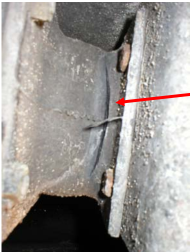
Fig. 4. Condition 2 - Tear 1-inch to 3-inches Wide, Across the Shear Spring, 1/4-inch Deep
